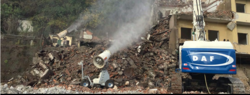
CIVIL AND INDUSTRIAL DEMOLITIONS
